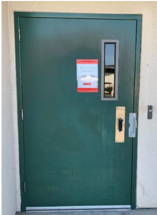
West facing Operations door
